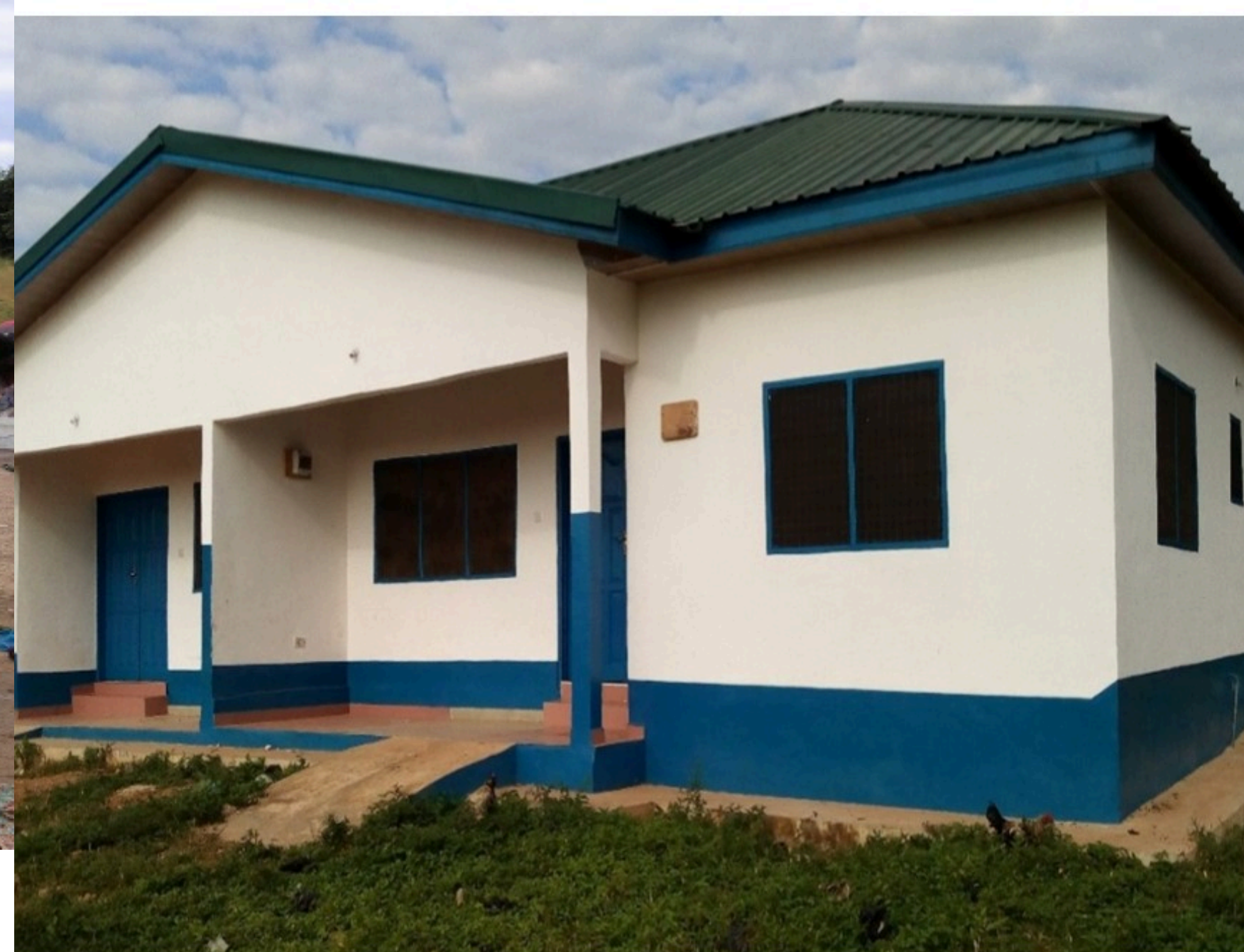
TEACHERS QUARTERS WITH MECHANISED BOREHOLE @ NYINAWUSU
