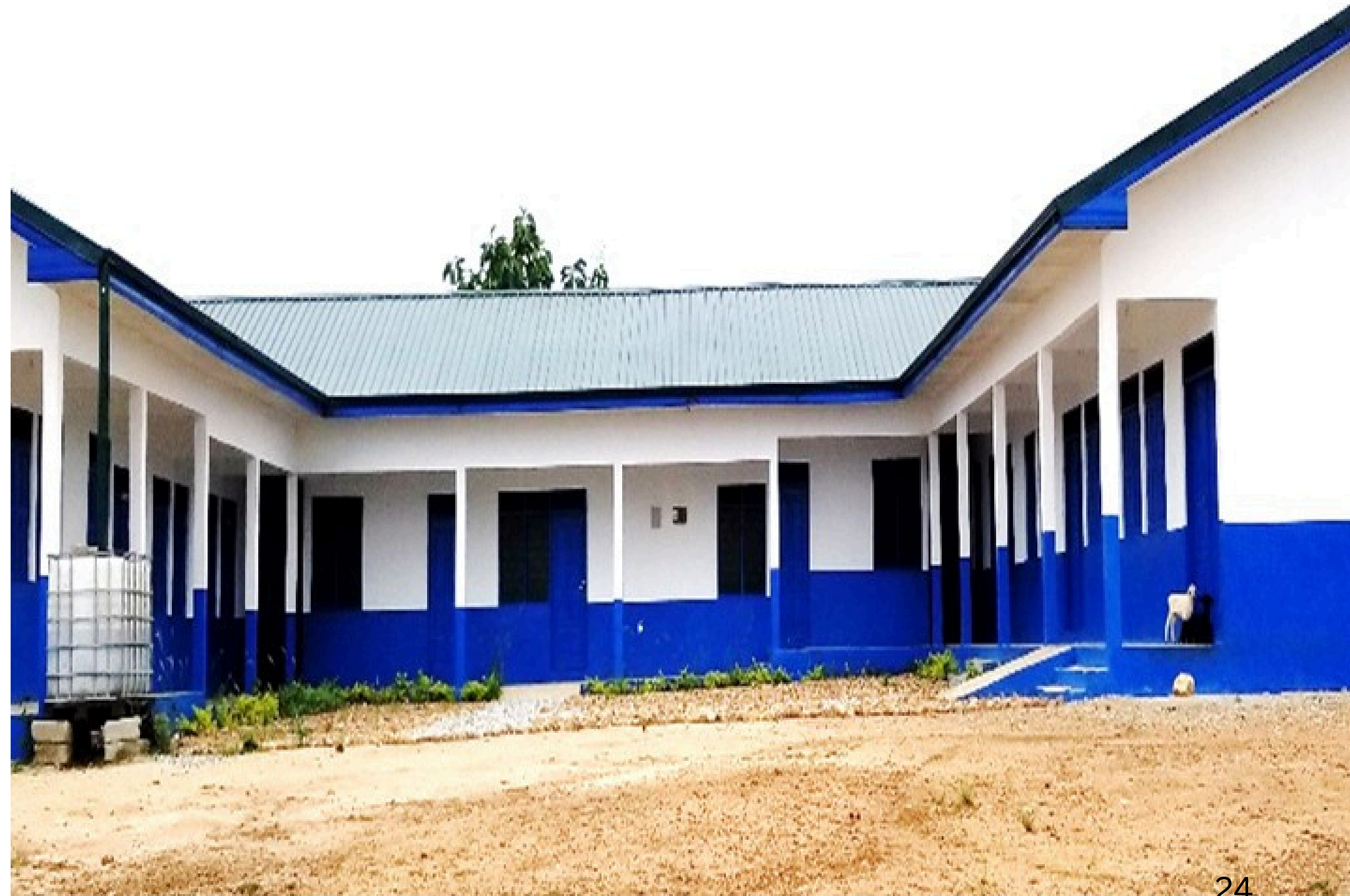
6-UNIT CLASSROOM BLOCK WITH 8-SEATER LATERINE AT EGYIRIFA
