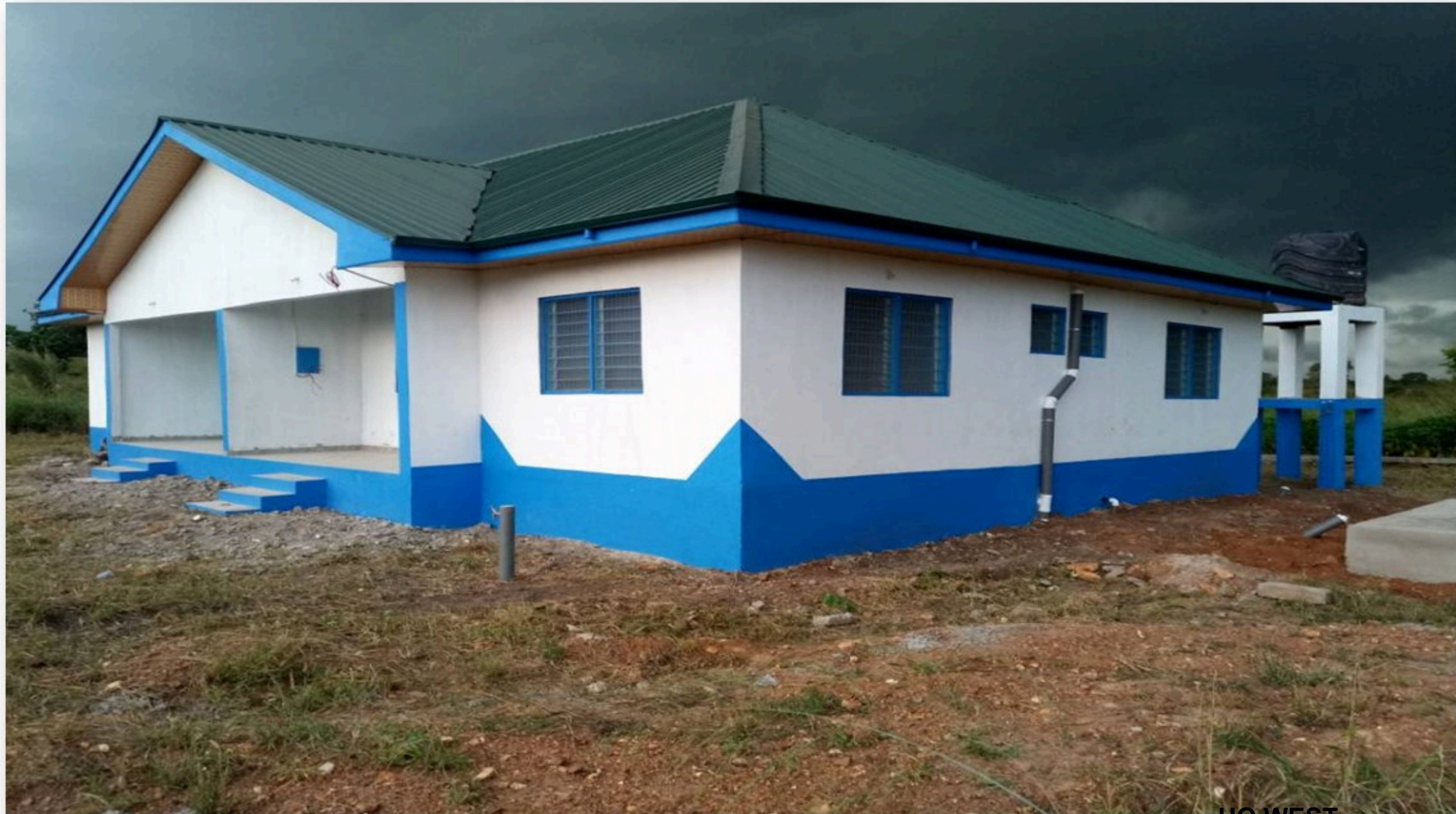
NURSES' QUARTERS WITH MECHANIZED BOREHOLE AT ABUTIA KISSIFLUI - HO WEST
