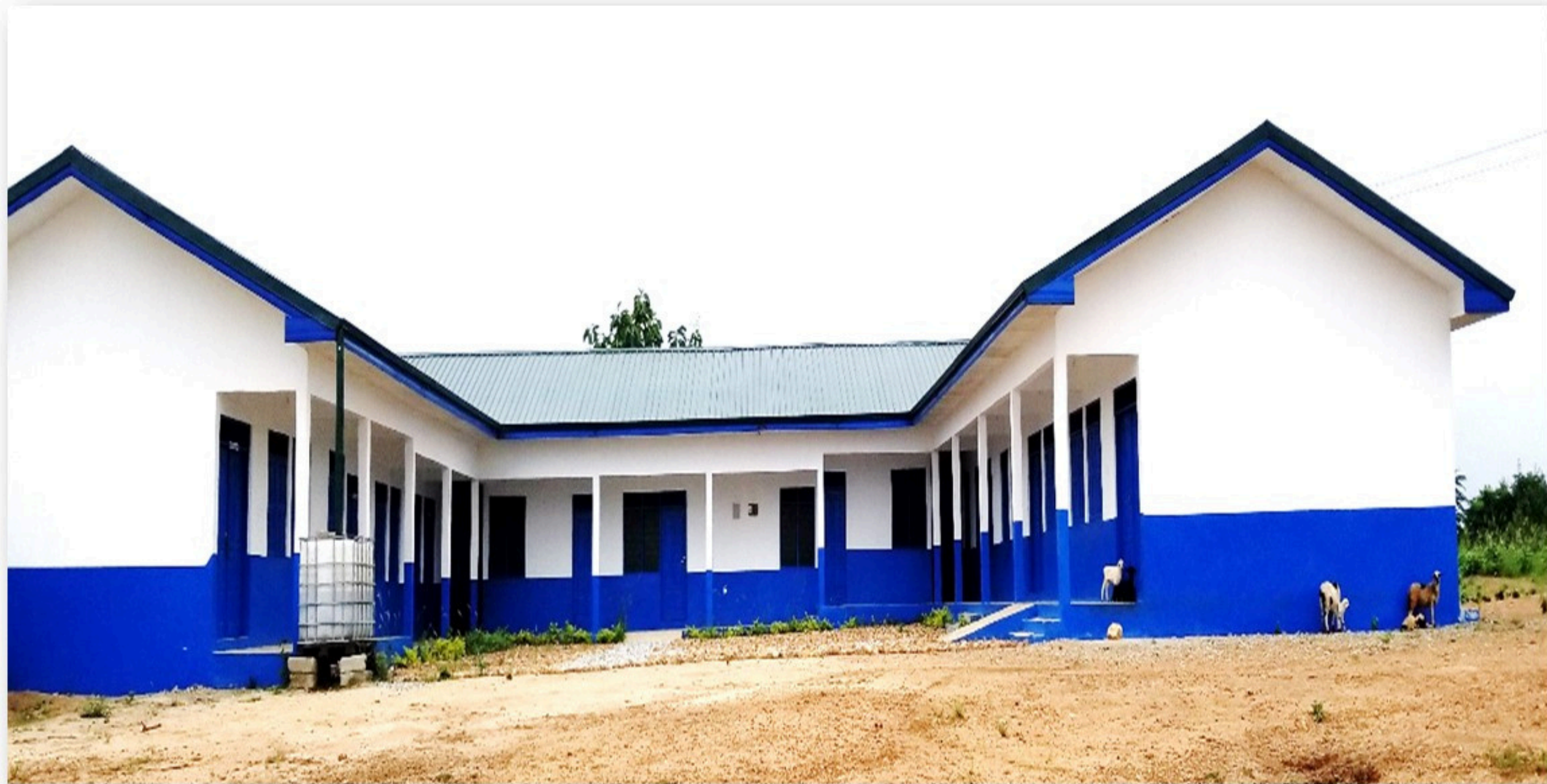
6-UNIT CLASSROOM BLOCK WITH 8-SEATER LATERINE AT EGYIRIFA
