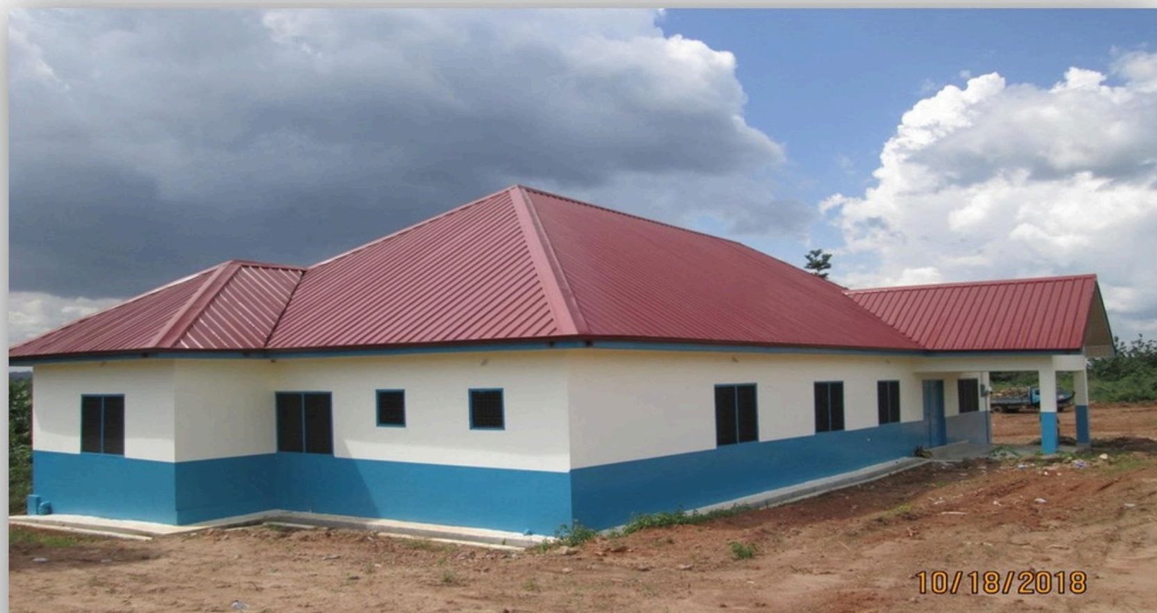
RURAL CLINIC WITH BOREHOLE AT NKWANTANAKESE
