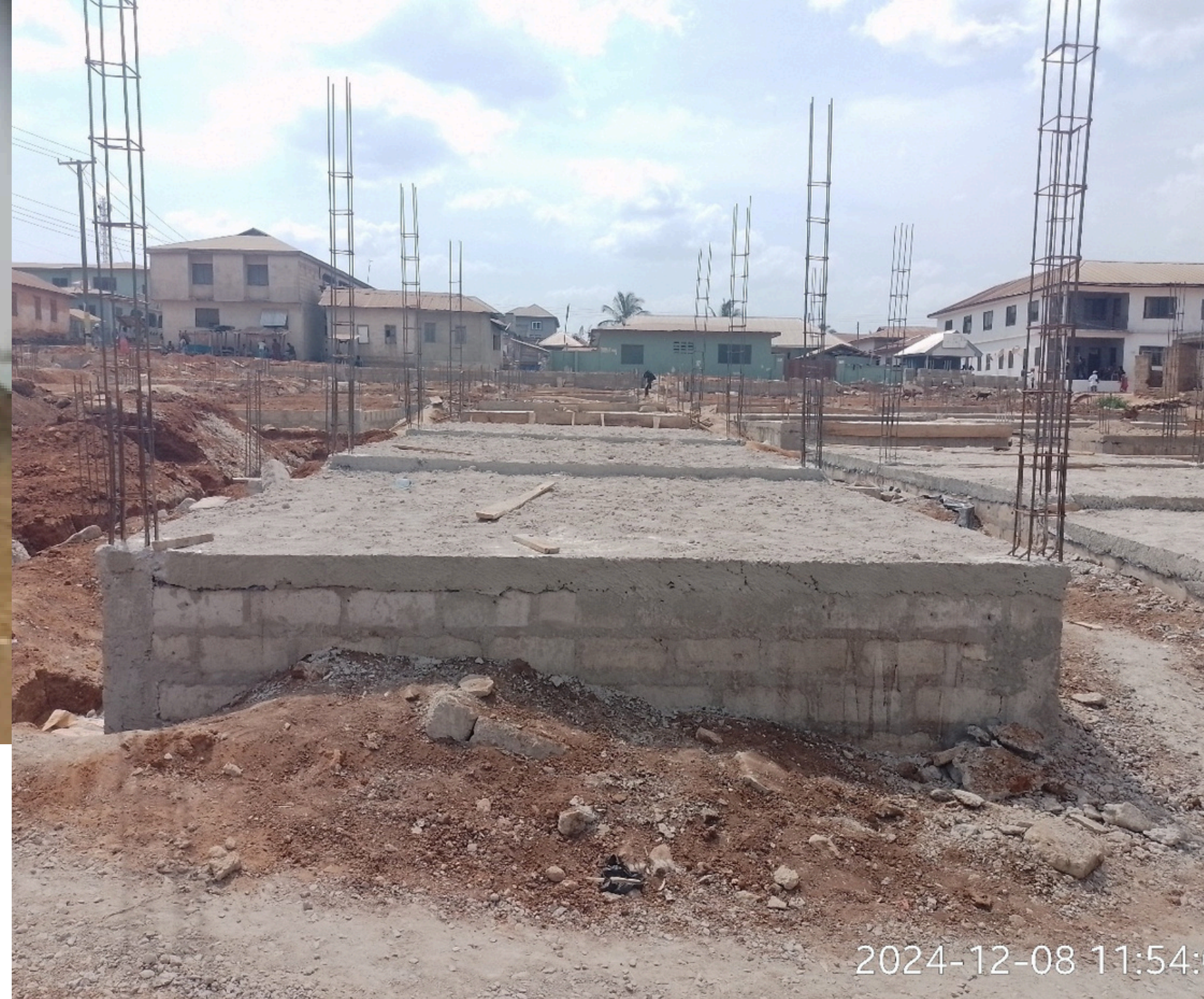
Construction of a Market at Beposo in Sekyere Central District
