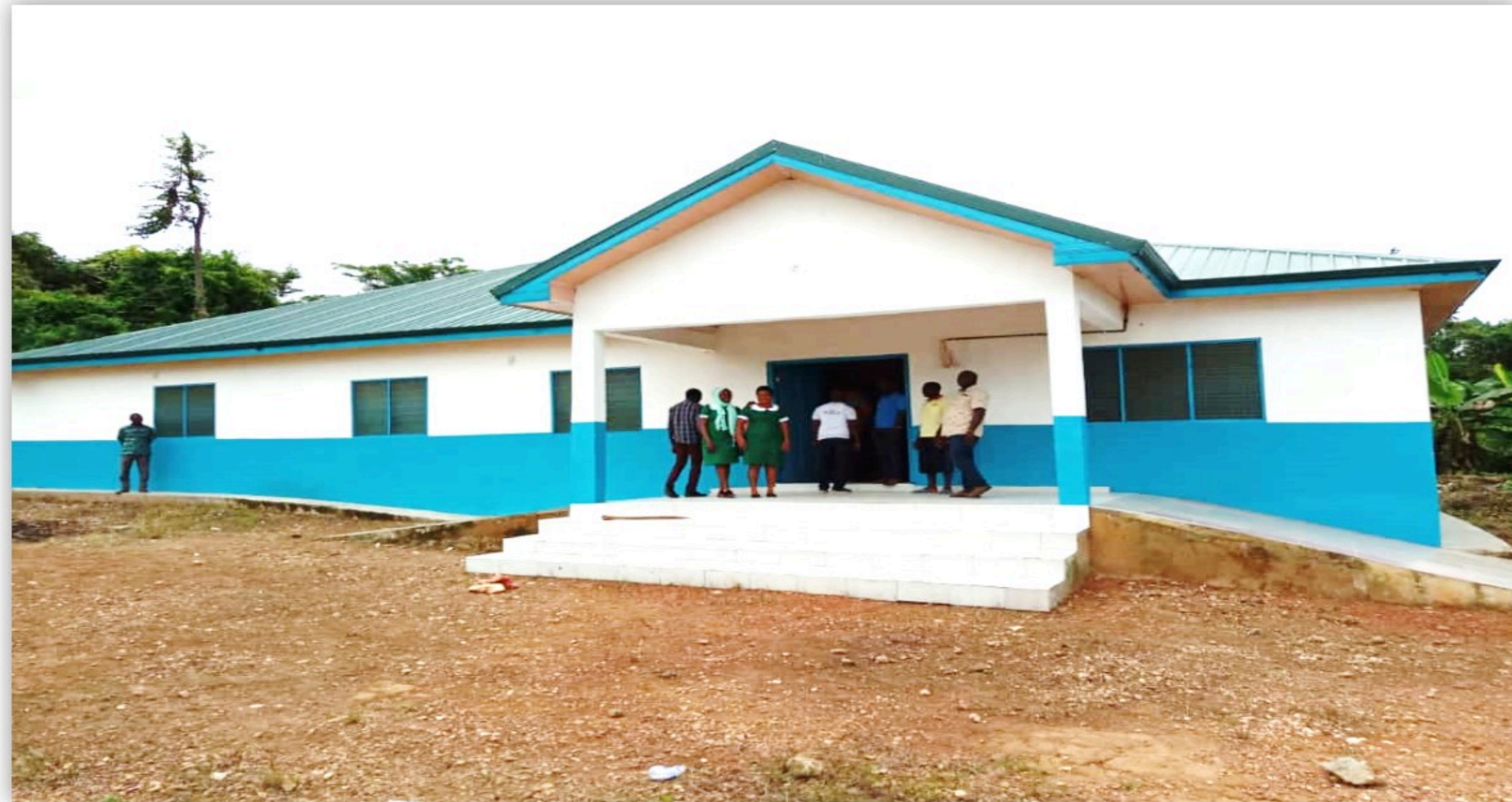
RURAL CLINIC WITH MECHANIZED BOREHOLE AT NKOTOMSO
