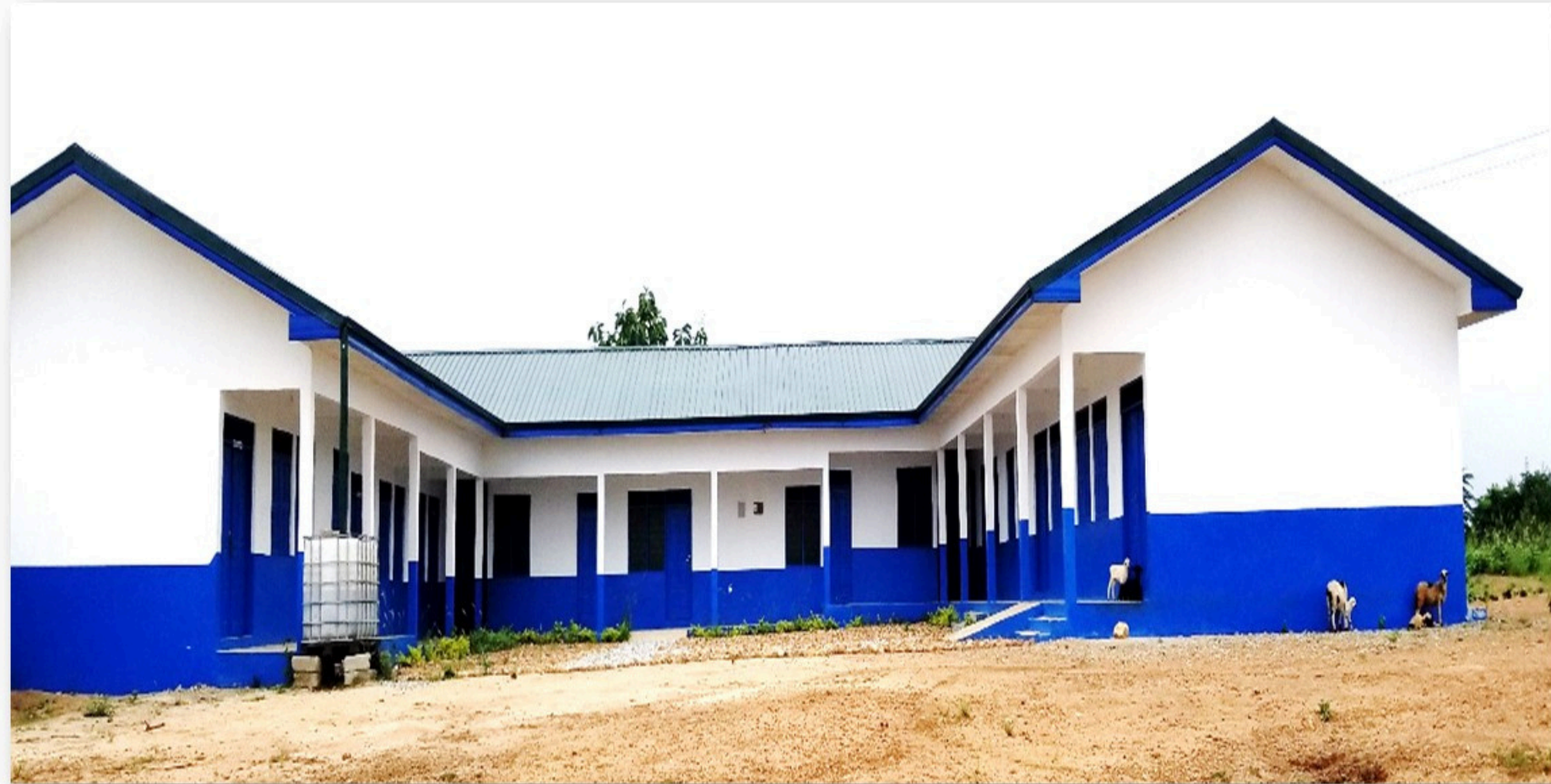
6-UNIT CLASSROOM BLOCK WITH 8-SEATER LATERINE AT EGYRIFA
