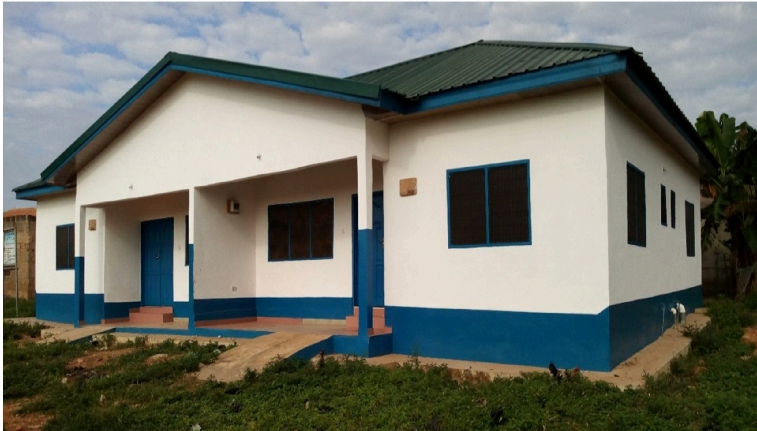
TEACHERS QUARTERS WITH MECHANISED BOREHOLE @ NYINAWUSU
