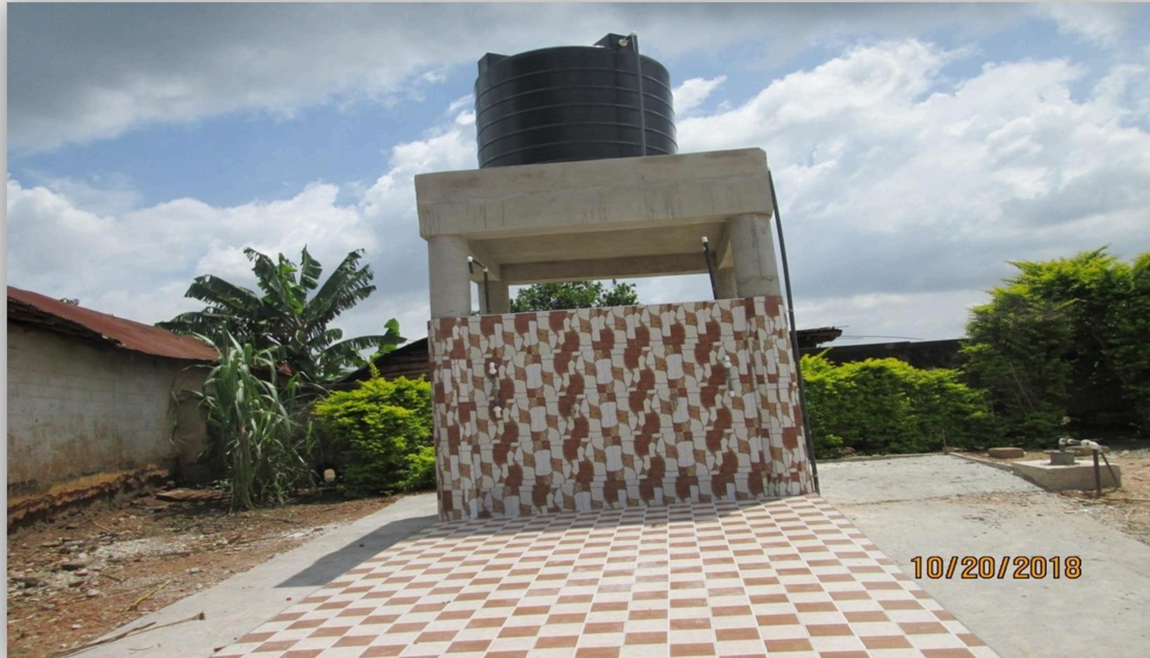
COMMUNITY MECHANIZED BOREHOLE AT WAWASE
