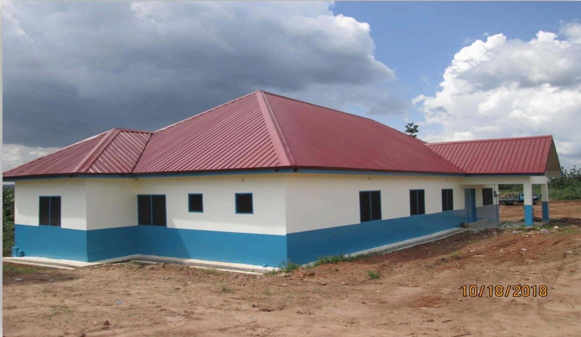
RURAL CLINIC WITH MECHANIZED BOREHOLE AT NKWANTAKESE - AFIGYA KWABRE
