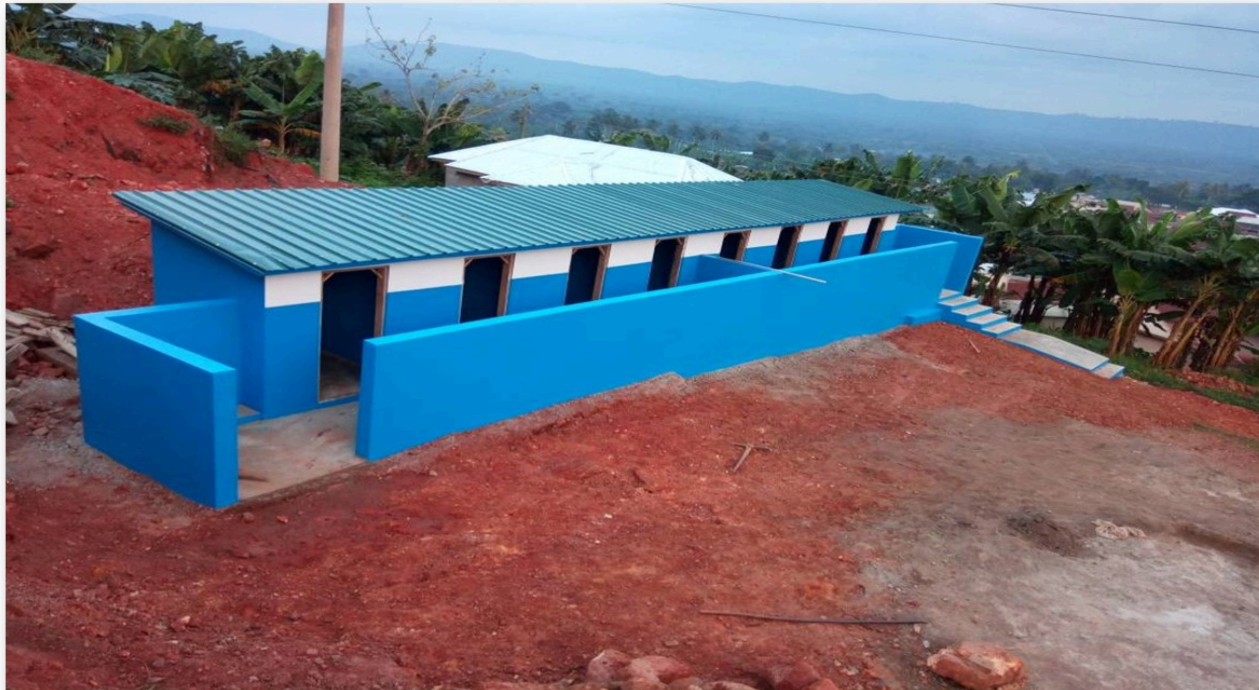
8-SEATER KVIP ATTACHED TO THE 6-UNIT CLASSROOM BLOCK AT TSITO
